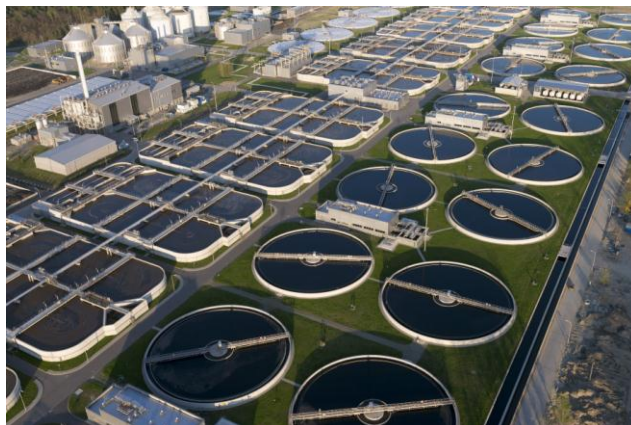
Czajka Wastewater Treatment Plant.
